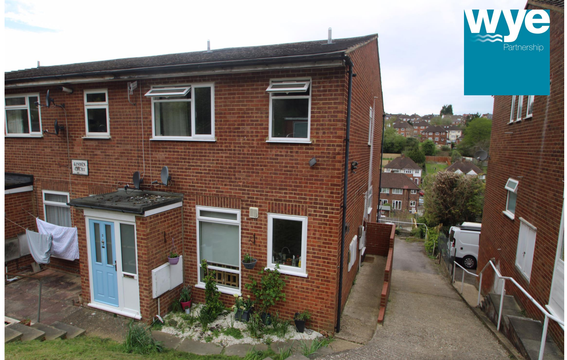
Carrington Road, High Wycombe, Buckinghamshire, HP12 3JB
